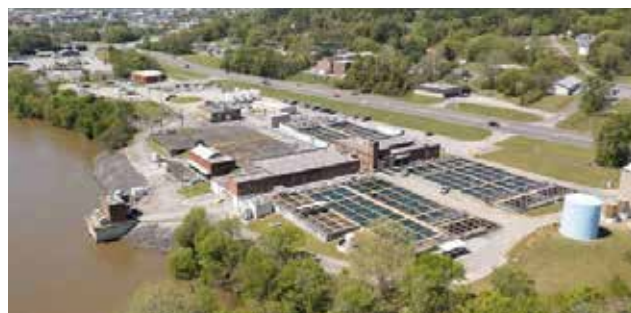
GADSDEN WATER TREATMENT PLANT
